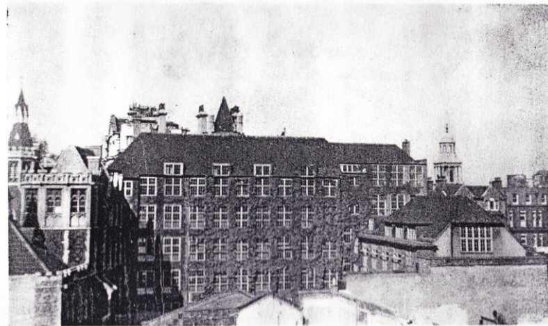
A VIEW OF THE SCHOOL DURING DEMOLITION OF ADJACENT SITE
